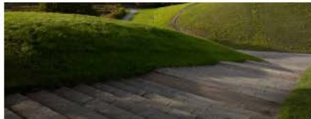
CONCRETE KERB AND BREEDON GRAVEL STEPS UP TO TOP OF CENTRAL FEATURE MOUND
